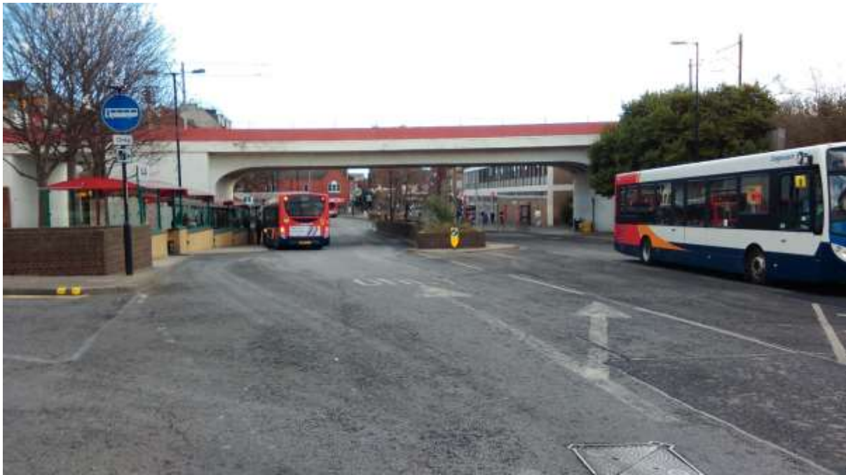
PLATE 7: VIEW EASTWARDS ALONG KEPPEL STREET TOWARDS FOWLER STREET JUNCTION
